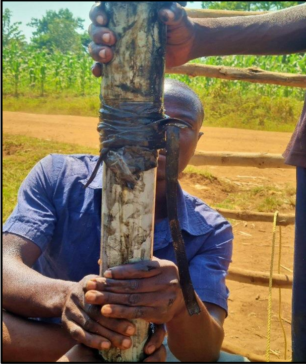
The plastic pipes and cylinder were replaced with resilient stainless-steel material.
