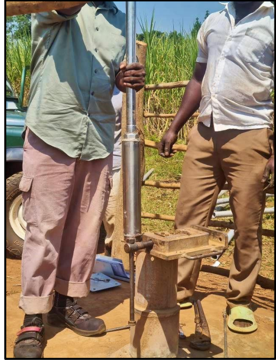
The plastic pipes and cylinder were replaced with resilient stainless-steel material.
