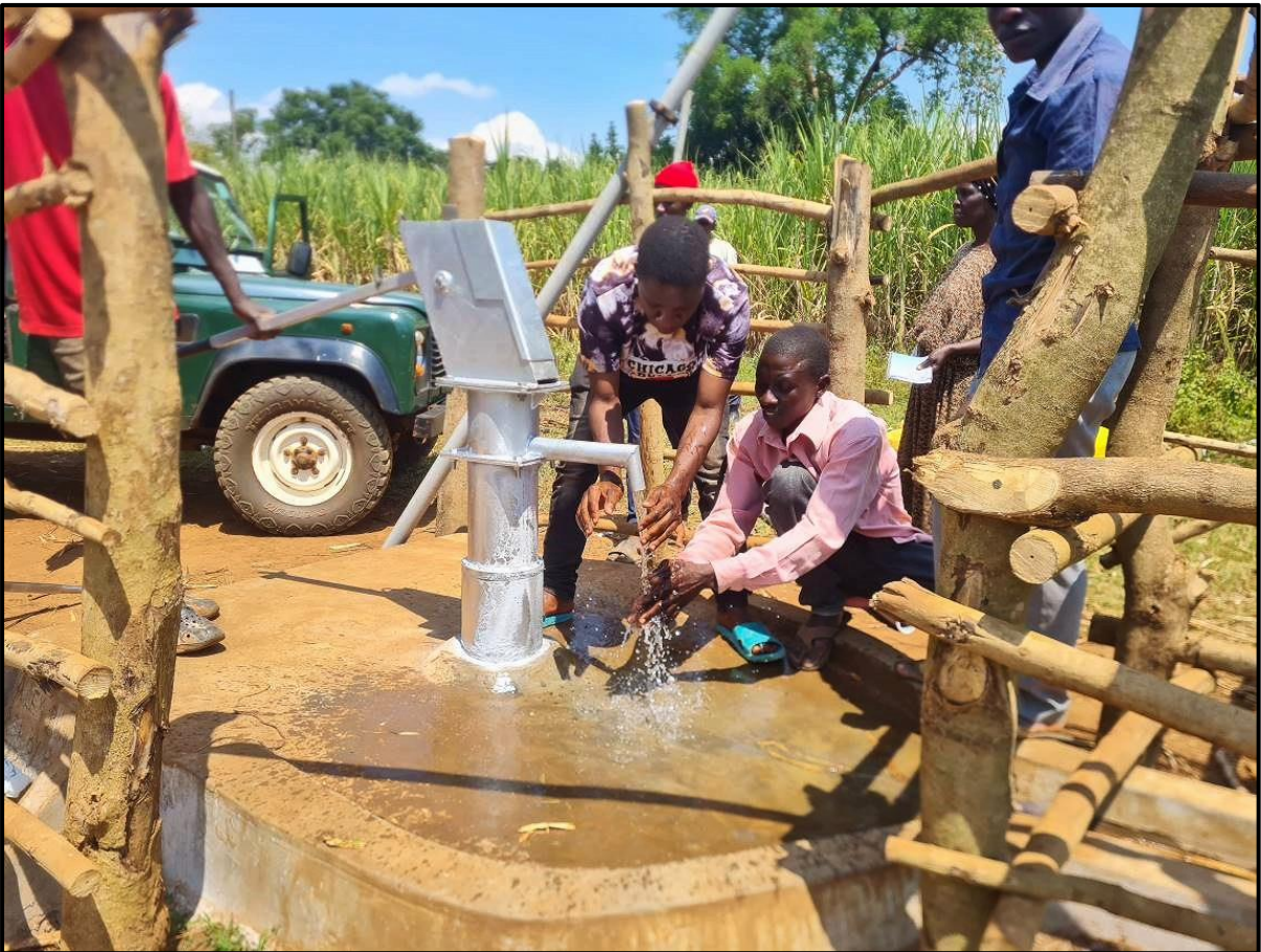
Flowing water after the rehabilitation of the Buwooya Alexander borehole.
